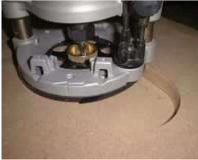
Locate template #2 on actual speaker baffle to route out the recess for the driver plate. Be aware that template #2 is  $\frac{1}{4}$ " wider around the perimeter of the driver plate. The depth will vary with the flange depth of the speaker driver.
